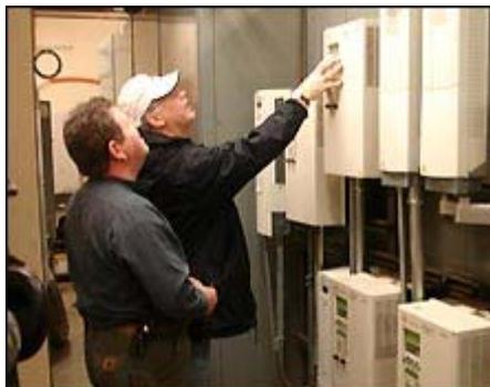
Variable frequency motor speed controls can be easily applied to fans, pumps and blowers, making them ideal for use on heating, ventilating and air conditioning systems.
