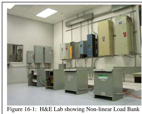
Figure 16-1: H&E Lab showing Non-linear Load Bank
